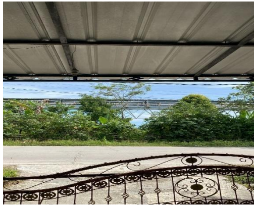
Figure 2. Proximity of the Factory Conveyor Belt to a Residential Area, showing the proximity of noise sources and material pollution.
